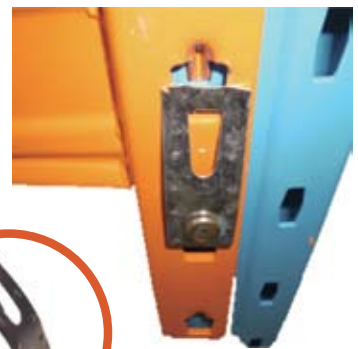
Check beam slots on the upright.
